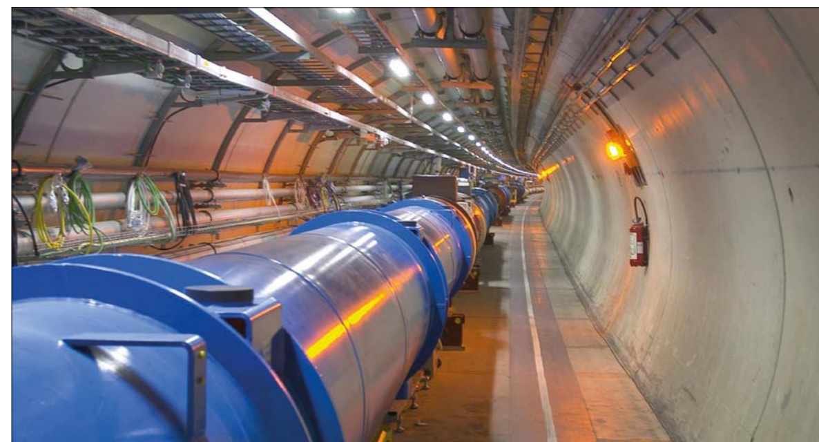
The first magnets installed in the LHC tunnel, in April 2005. The last of the 1232 dipoles was put in place two years later.
